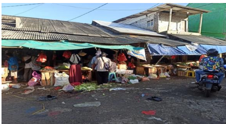
Figure 1.3 Road narrowing at Surade Traditional Market (Source: Surade Market, 2021)
