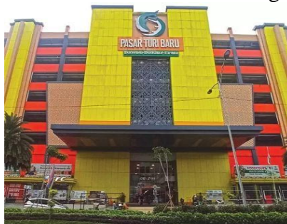
Figure 1. Front view of the Pasar Turi Baru
